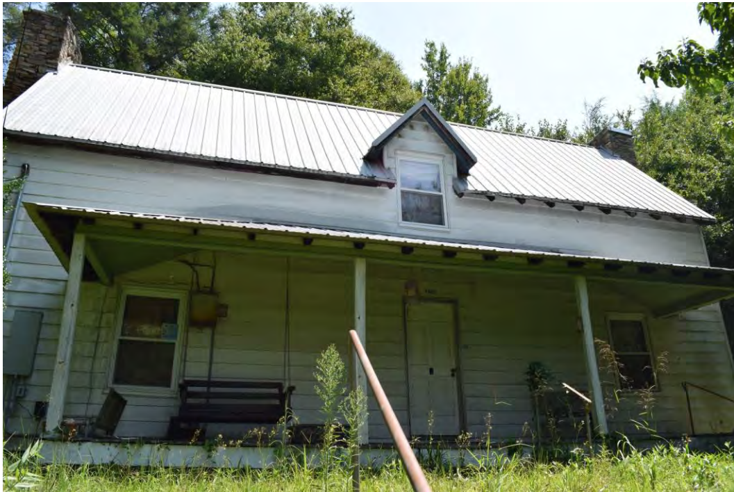
Facade, view to the east
