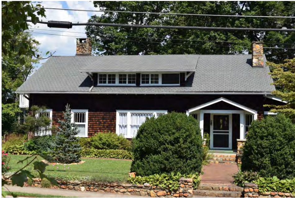
Rev. C.D. Chapman House, view to the northeast
