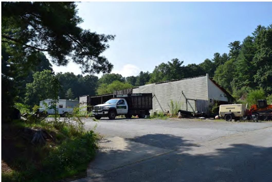
Maintenance Buildings #2 (left) and #1 (right), view to the southwest
