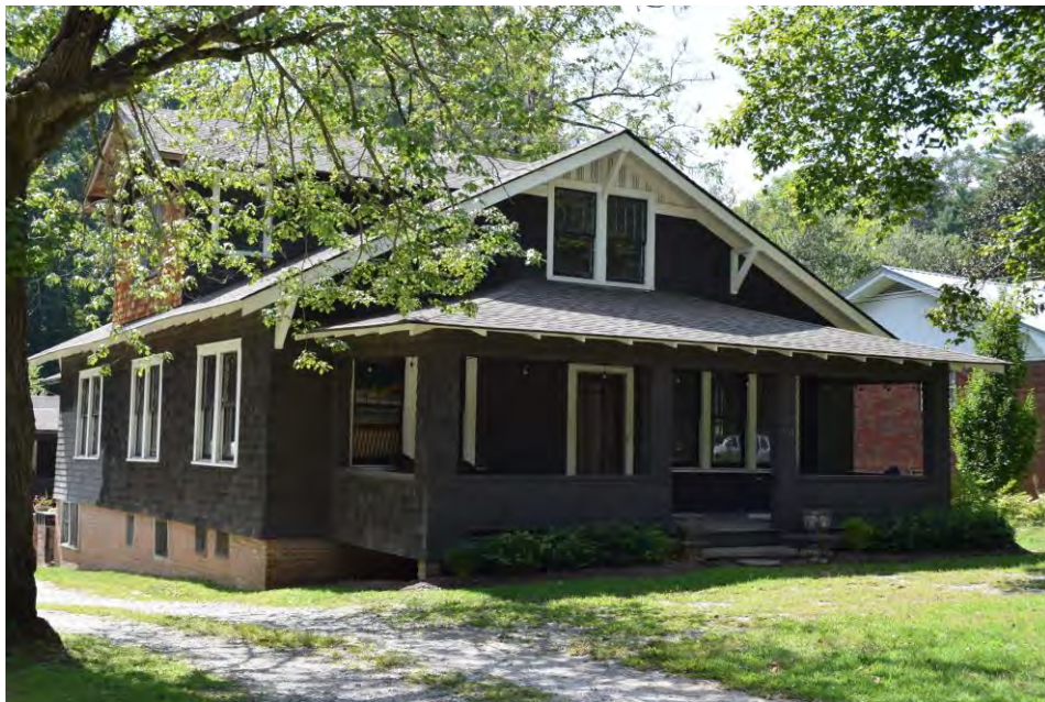
Shingled bungalow at Lingerlong Apartments, view to the northwest
