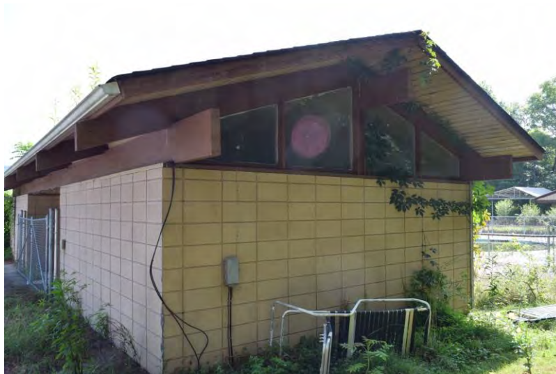
Pool changing rooms, view to the south
