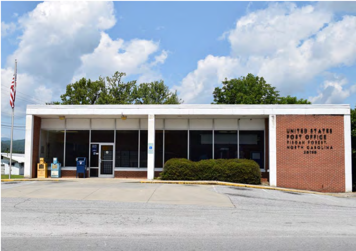
Façade (southeast elevation), view to the northwest
