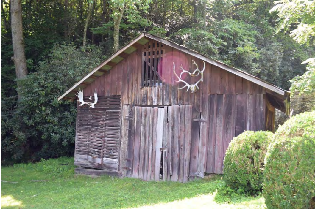
Barn/corncrib from circa 1925, view to the northeast
