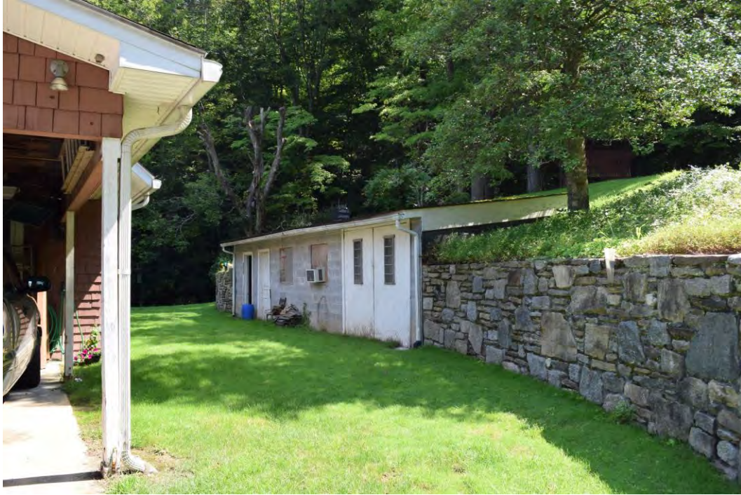
Bank house and modern stone wall, view to the north-northeast
