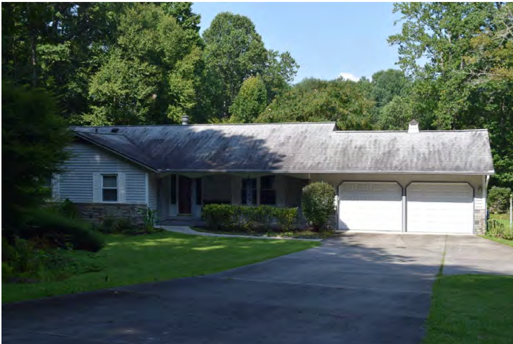
House, 1507 Glen Cannon Drive, 1975, view to west
