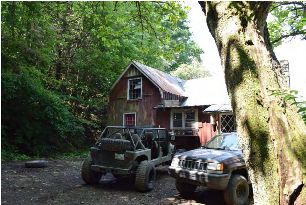
Rear elevation, view to the west-southwest
