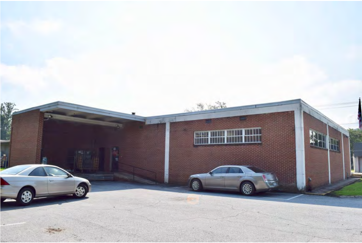
Rear elevation, view to the southeast
