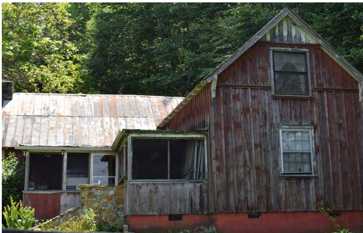
Facade, view to the east
