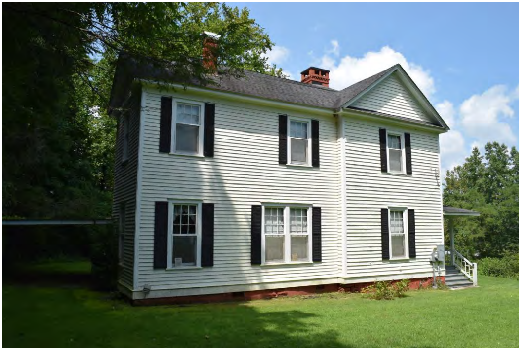
Jenkins House, east elevation, view to the west-northwest
