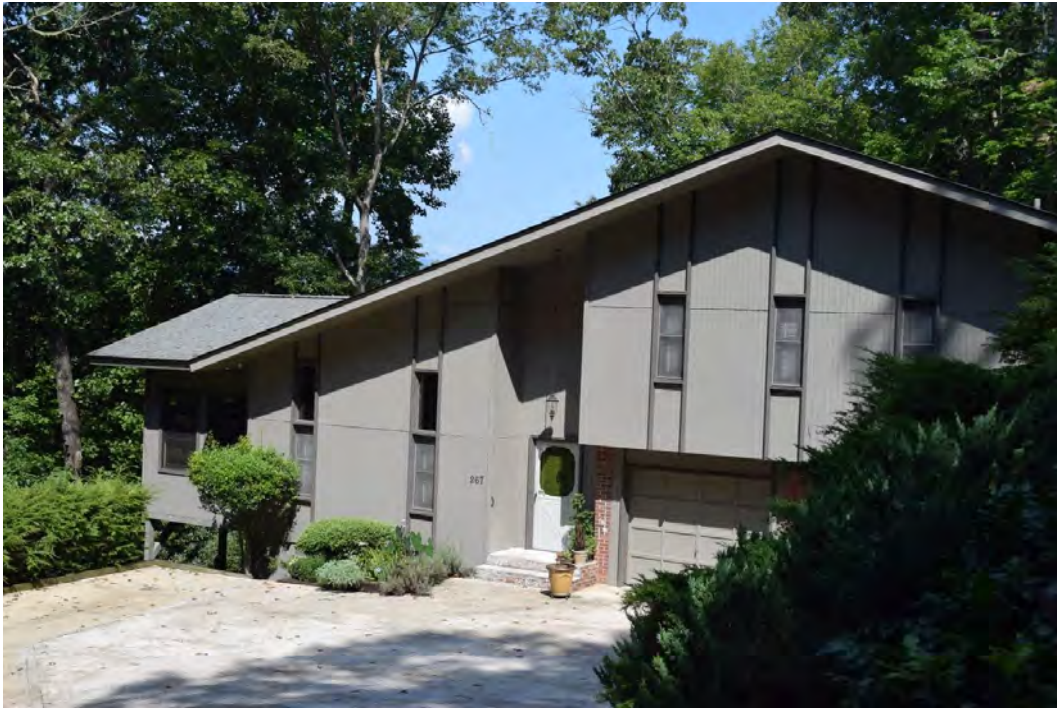
House, 267 Campbell Drive, 1978, view to southwest
