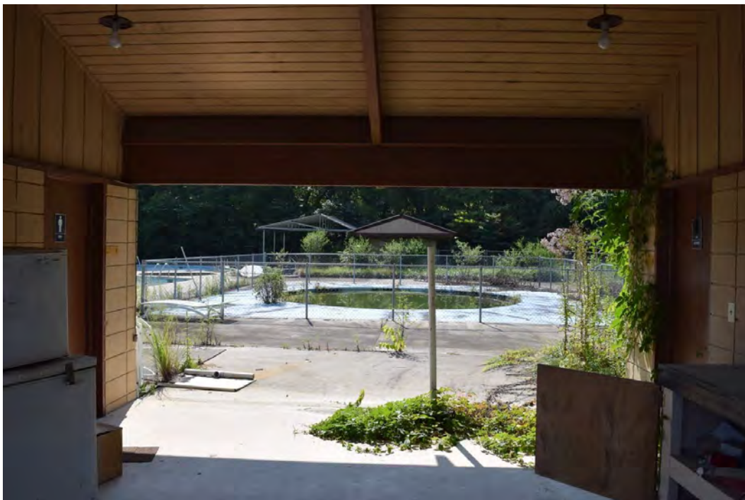
View to the pools through the changing rooms with poolhouse in background, view to the east
