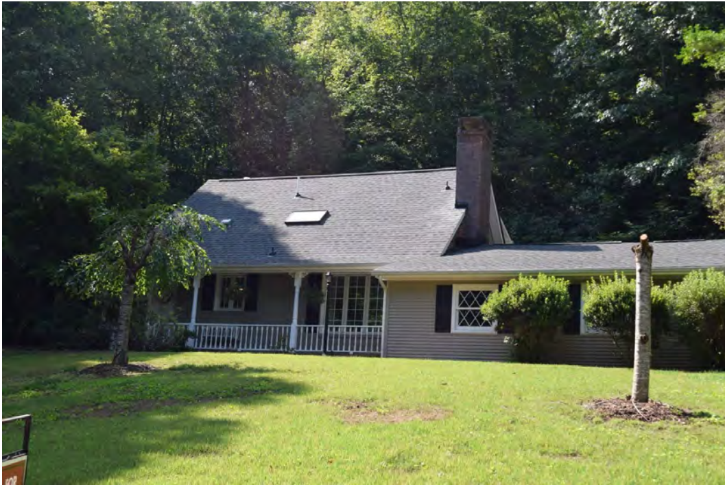
House, 1134 Glen Cannon Drive, 1973, view to south
