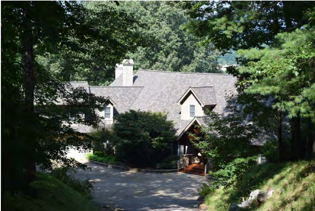
House, 1303 Glen Cannon Drive, 1992, view to west
