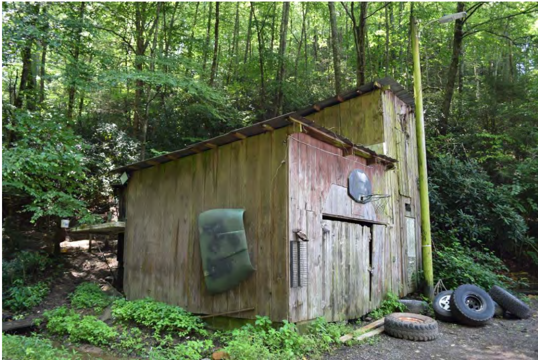
Springhouse and shed, view to the south
