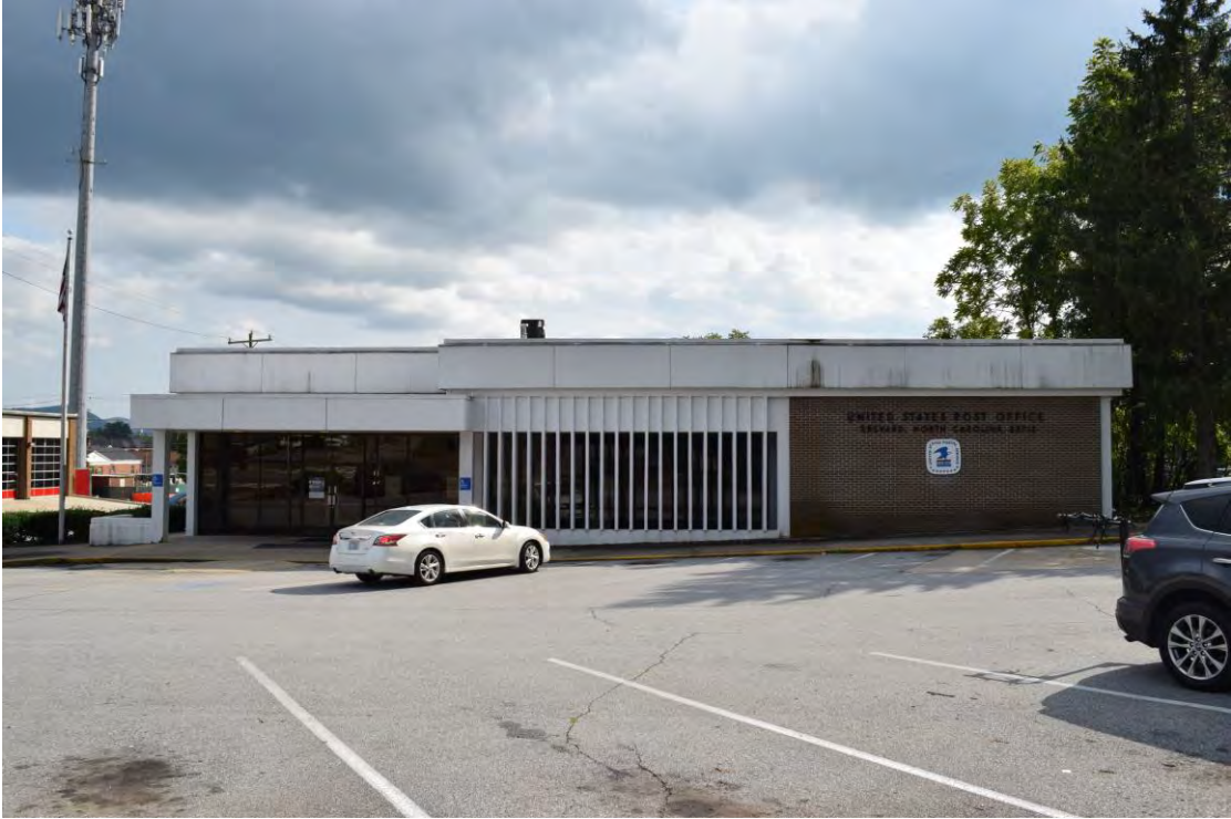
Brevard Post Office, 1972, view to the south
