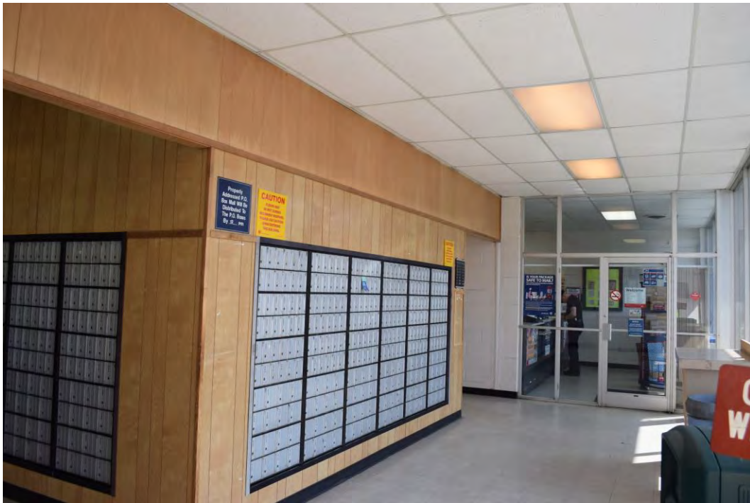
Lobby looking into the retail area, view to the northeast
