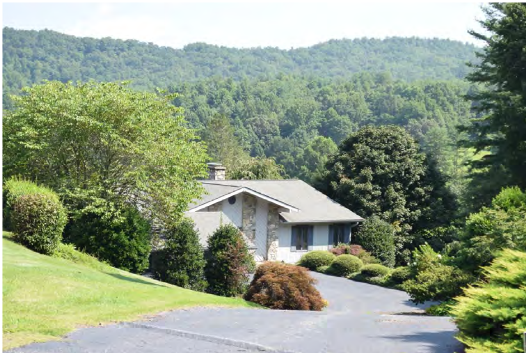
House, 82 Douglas Circle, 1982, view to northeast
