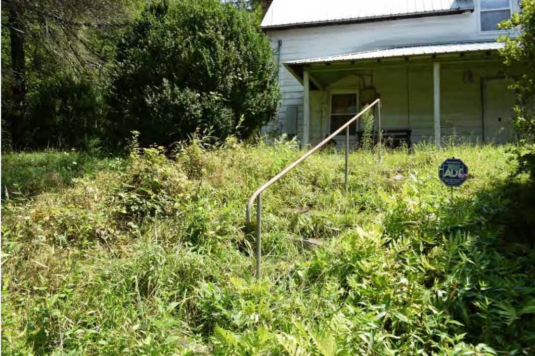
Overgrown concrete steps leading to the front of the house, view to the northeast
